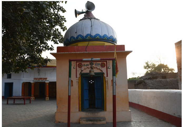
Figure 4 : Shiva Temple, Mujaffarnagar, Sahawar Tehsil Source: Primary survey by AH Division, INTACH Team
