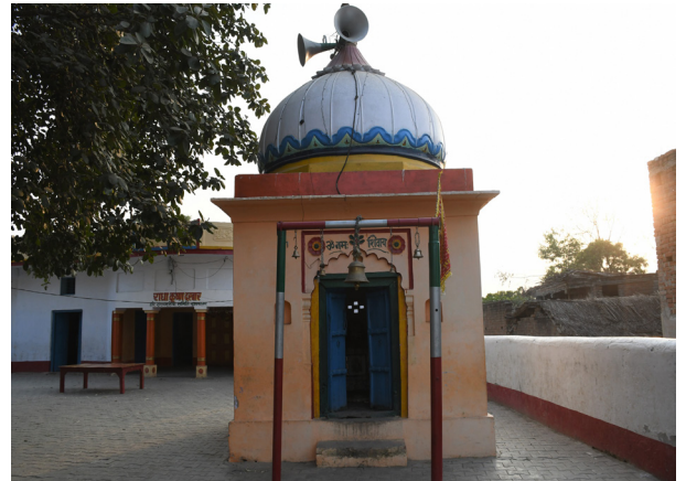
Figure 18: External facade of the Shiv Temple Source: As per primary survey done on site
